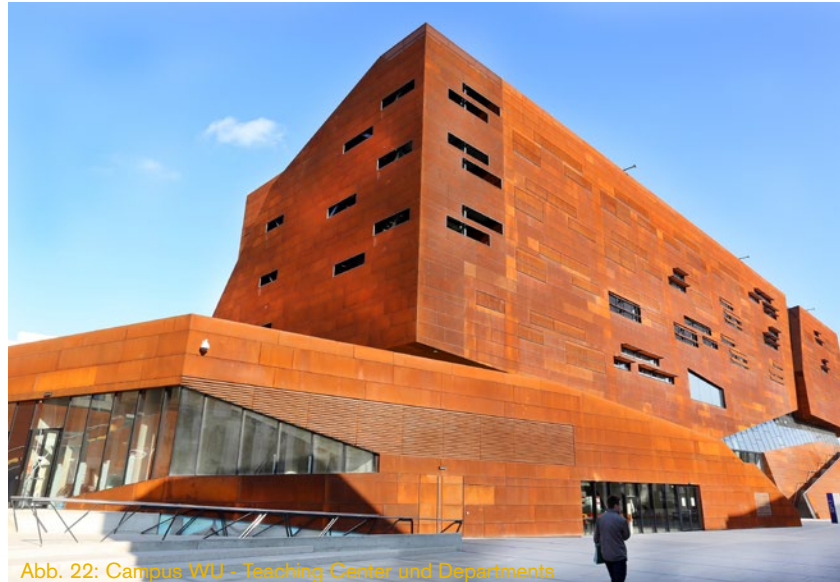
Abb. 22: Campus WU - Teaching Center und Departments
